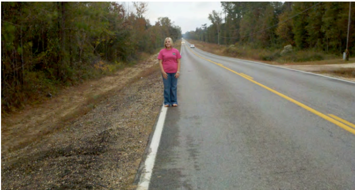
A Southeastern Louisiana University student has “Found the Fault” on LA Highway 441 (Used by permission).
