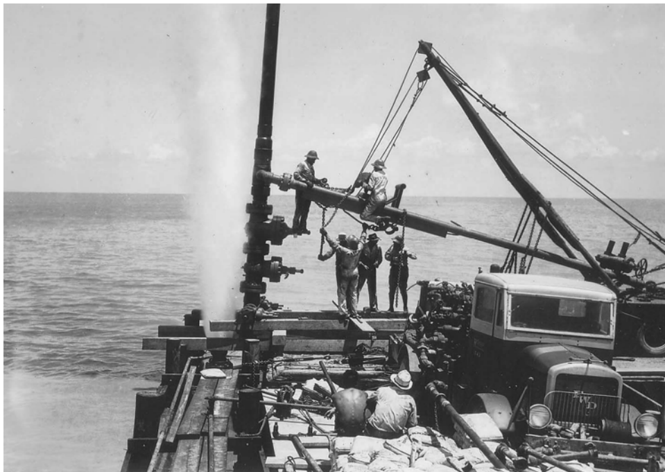
Figure 4. Working on a Blowout.
