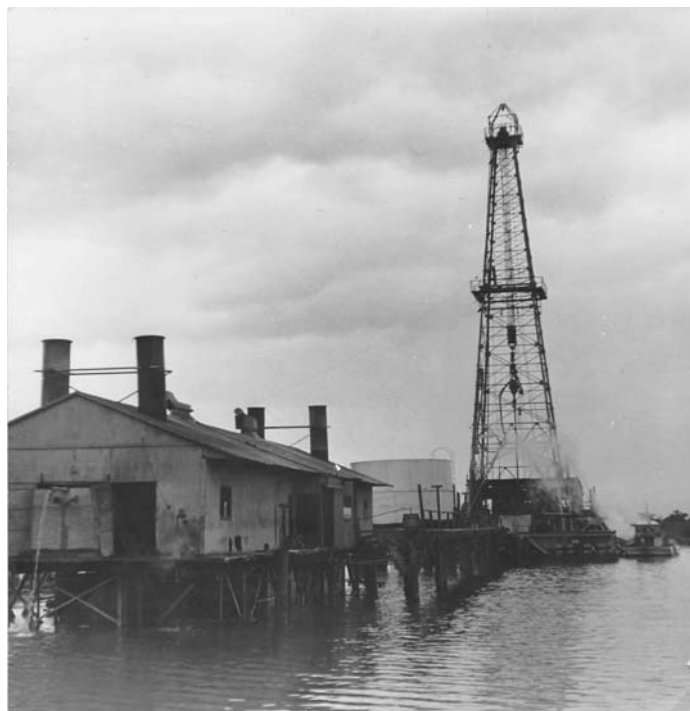
Figure 10. Barge Drilling Rig by Field Facilities.
