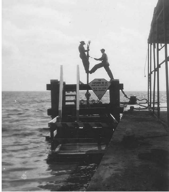
Figure 15. Men Working on a Well.
