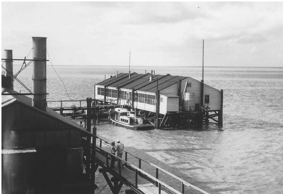
Figure 14. Field Office Complex.
