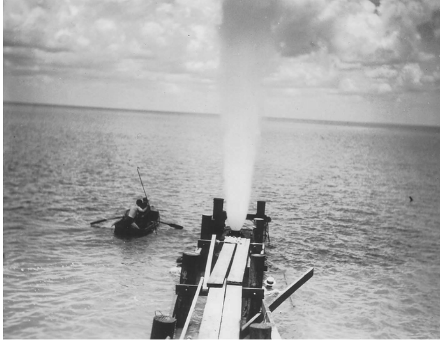
Figure 3. Assessing a Blowout.
